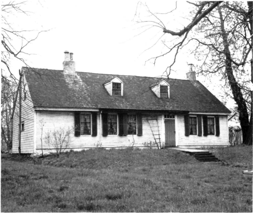
9. The north front in 1947. Note the horizontal window and plumbing stack on the east end, (left hand side) and the Victorian Gothic Chimney Pots. The overall deformation of the house can be seen by the drooping ends.
