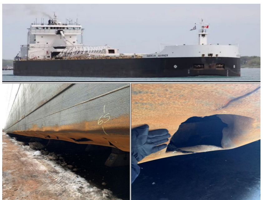
Fig. 7 Damage to the port water ballast tanks of bulk carrier American Merine due to grounding (Source: US Coast Guard).
