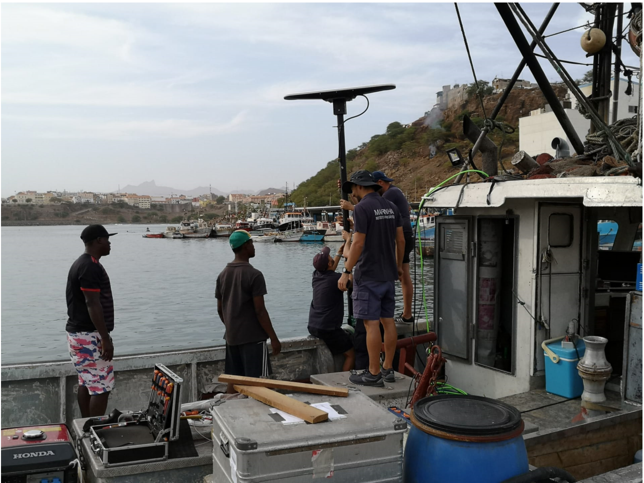
Figure 7. Multibeam installation in a vessel of opportunity.
