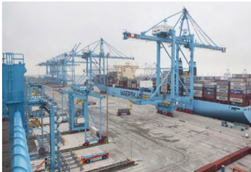
Figure 4. Maasvlakte II Terminal at Port of Rotterdam
