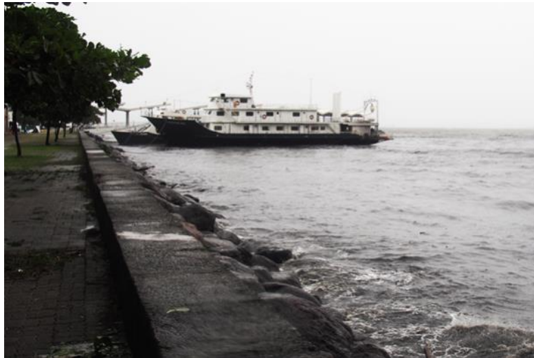
Figure 13. Behind the breakwater in Figure 11 (15 September 2018). Waves do not form behind the breakwater
