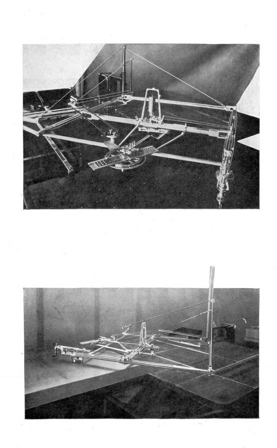
connecting rod, is controlled by an adjustable pivot-point fastened to the compensating bar. The pivot point is free to move longitudinally between rails which are rigidly held in place so as to prevent any lateral movement of the pivot-point to the right or left. The copy-board is mounted on ball bearing rollers so as to permit any right or left movement transmitted to it through the compensating device.
