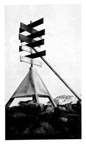
Type of signal recommended for mountain triangulation;  $2'' \times 2'' \times 8'$  pole,  $1/2'' \times 6'' \times 30''$  boards for lines of about 5 to 10 miles. The signal cloth around the three lower braces is not for pointing on, but merely to aid in picking up the signal easily. A round guy slightly above the middle of pole could be substituted for lower braces. The long brace prevents twisting of target in wind.
