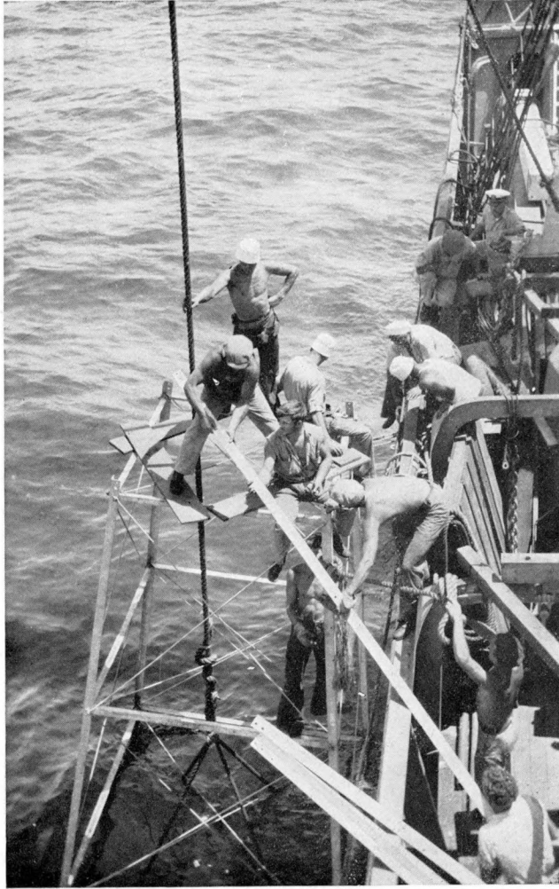
Completing Tower Suspended from Boat Boom.
