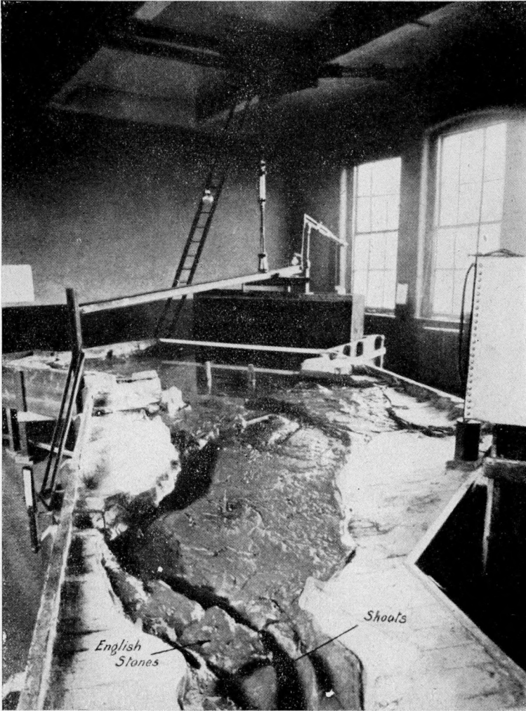
Fig. 2 Severn Model showing plunger.
