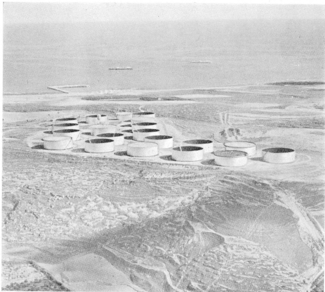
Photograph by Courtesy Trans-Arabian Pipeline Co.
