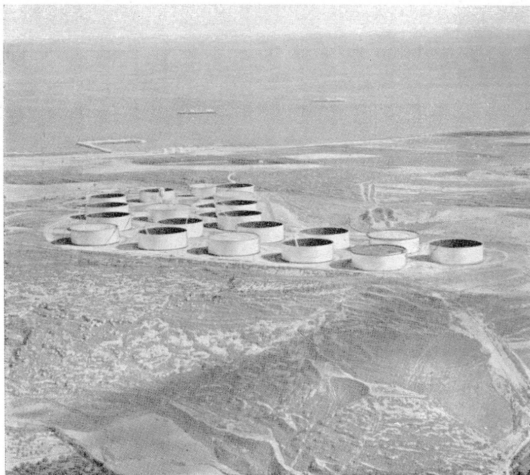
Photograph by Courtesy Trans-Arabian Pipeline Co.
