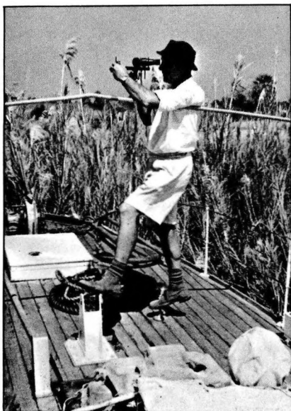
FIG. 9. — End of line. Lines of soundings were frequently carried right up to the shore. Commander TRIPP takes a sextant angle.
