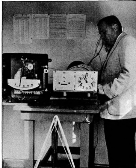
FIG. 4. — Standard Tide Gauge Installation with Remote Recorder.
