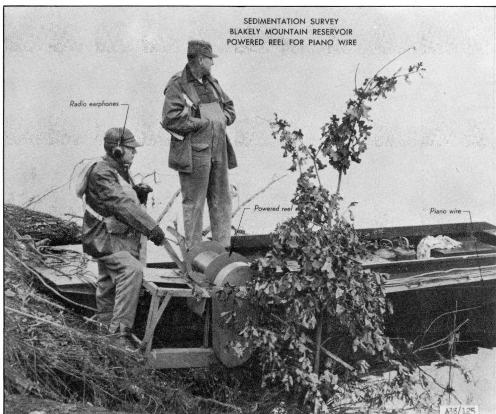
Fig. 3. — Powered Reel for Piano Wire
