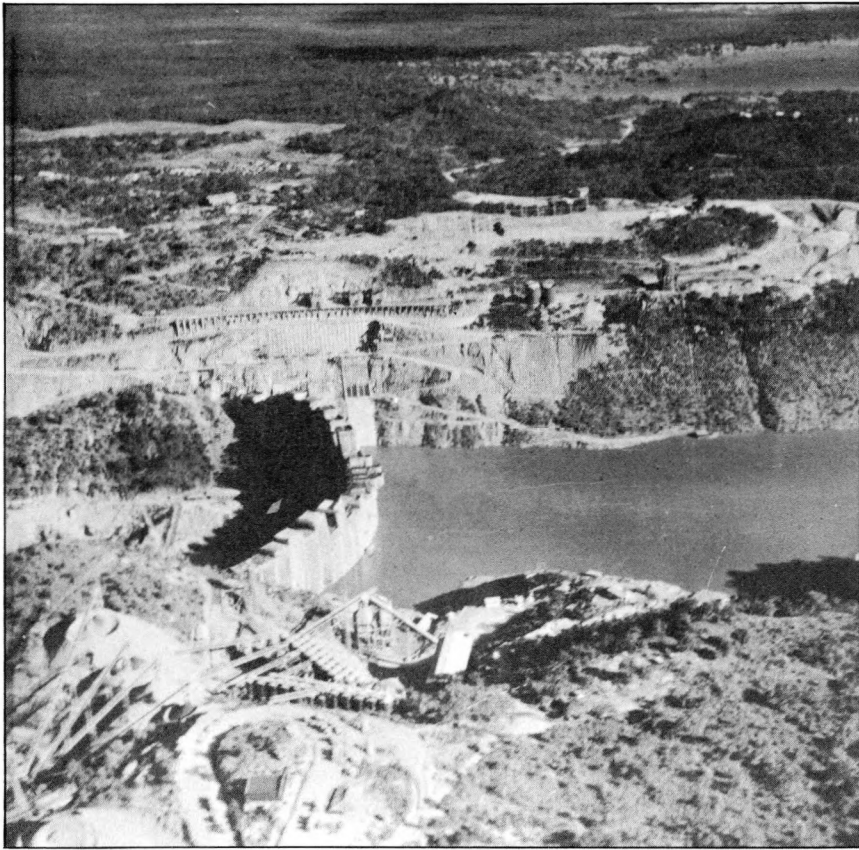
Fig. 2. — Aerial view of the dam in course of construction, showing the impounded waters of the Zambesi, Kariba township on the south side, and the new lake forming in the distance.
