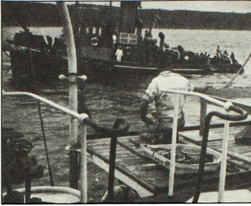
FIG. 3. — The operation of laying the undersea cable from the shore towards the wave recorder position. (Transducer assembly in foreground; target markers on shore visible over bow of boat).
