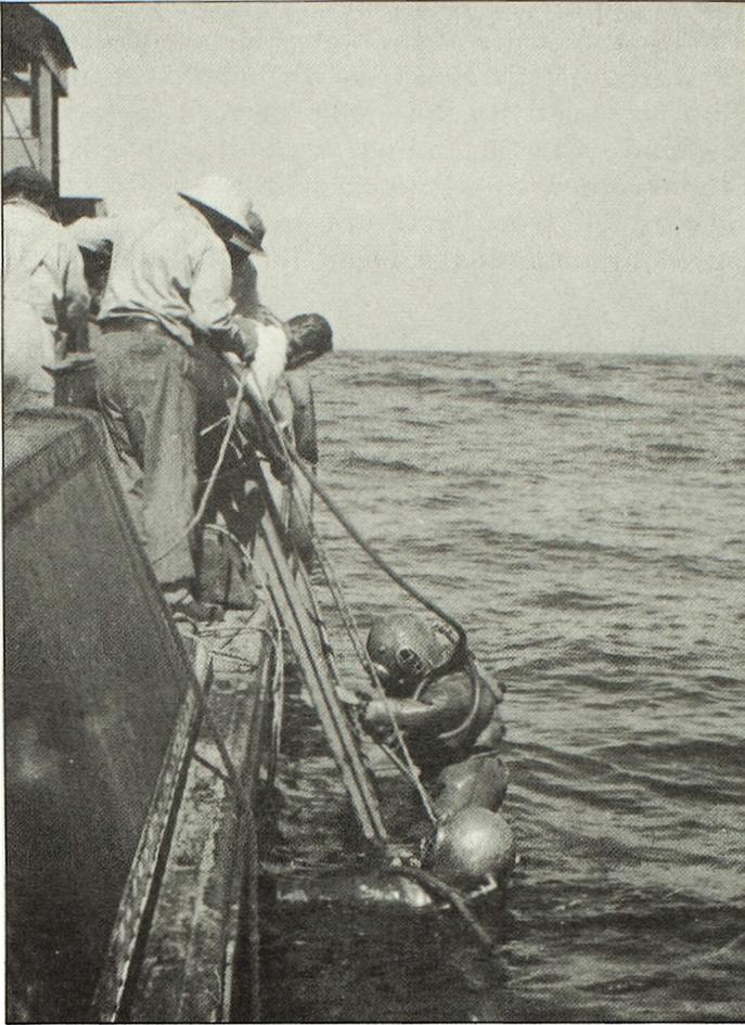
FIG. 6. — Divers going down to inspect and adjust stand two days after the recorder was placed.
