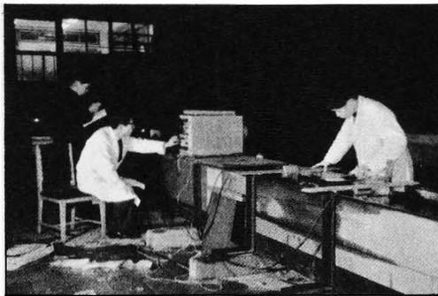
FIG. 13. — Measurement of transmission loss in ice.
