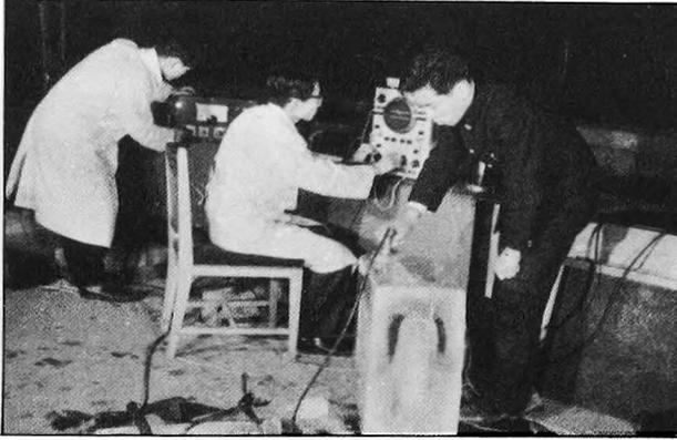
FIG. 16. — Measurement of sound velocity in ice.
