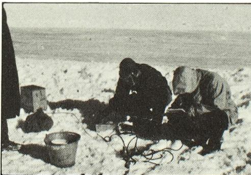
FIG. 8. — Sounding with two transistorized fish finders.
