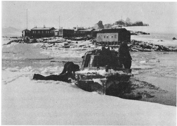
FIG. 4. — Carrying out temporary repairs to the survey boat after being holed by ice above the waterline. In the background is the British base on the Argentine Islands.
