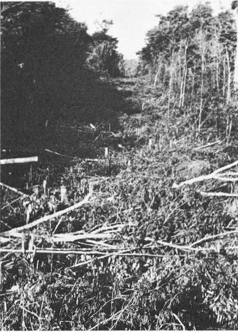
FIG. 2. — A path of about 10 metres wide had to be cleared.
