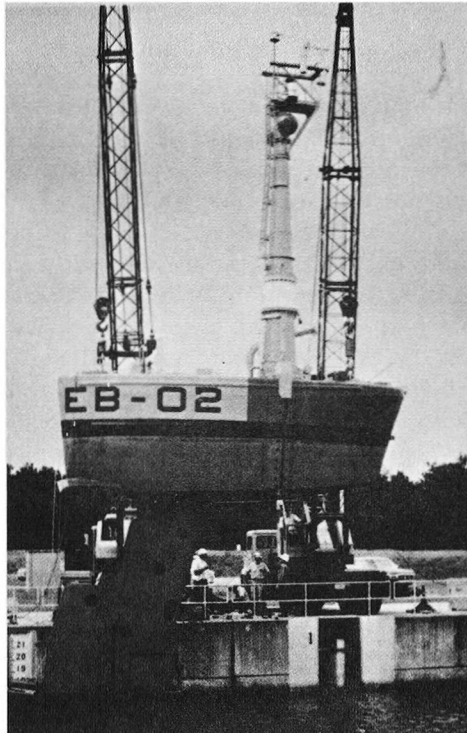
FIG. 12. — Deep keel hull environmental buoy.
