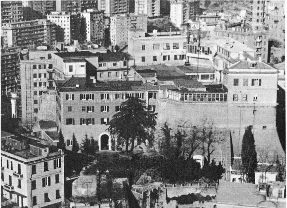
FIG. 2. — The Italian Hydrographic Institute in Genoa, formerly the old fort of St. Giorgio, a building it has occupied since its creation.
