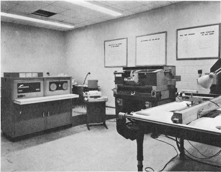
FIG. 3. — The Analytical Plotter Model AP/2C at the University of New Brunswick. From Left to Right — control computer of the system (interfaced with an IBM 360/50), teletype unit, viewer, and plotting table.
