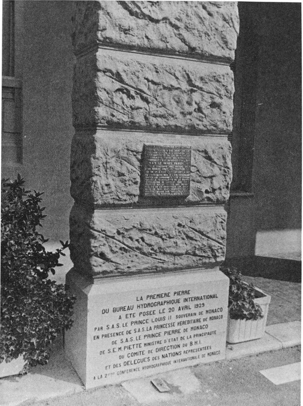
The bronze plaque above the Foundation Stone on the S.W. pillar of the IHB building. The bolt in the centre of the plaque marks its position in the World Geodetic System 1972.
