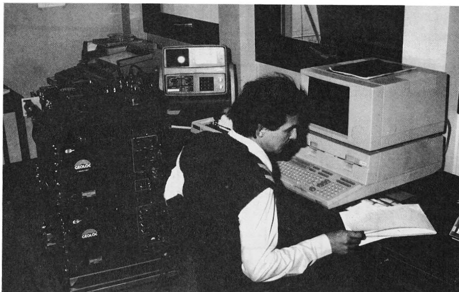
FIG. 9. — Typical mobile station. From left to right : Transit receiver, central processor, receiver and time keepers.
