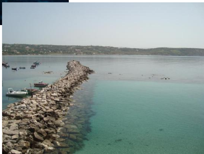
Figure 3. The 19 th century breakwater over the (nowadays submerged) ancient breakwater.
