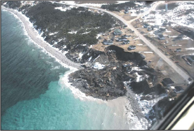
Figure 8. Landslide at Daniel's Harbour, Newfoundland. The slide was characterized as a combination of translational-slip failure and rotational-slip failure and occurred as a result of the saturation and subsequent loss of strength of a clay-rich layer underlying till.
