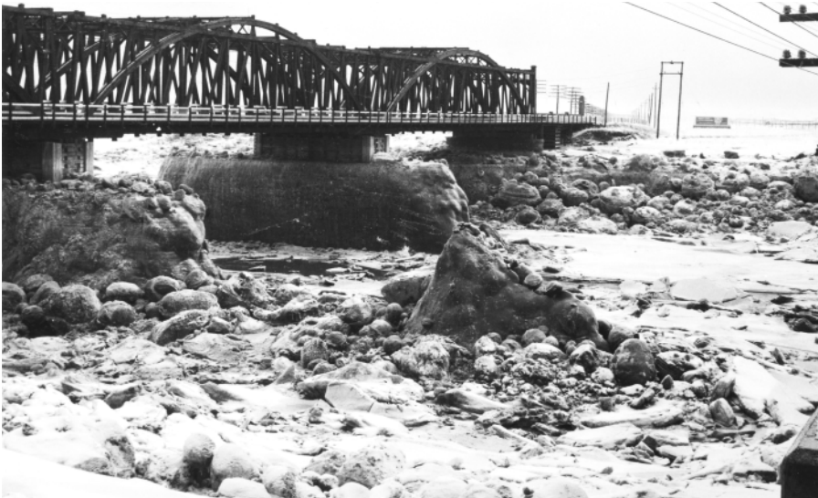
Fig. 53 Tantramar River downstream of former Highway 2 Bridge, Sackville, N.B., 12 March, 1959. Note the coating of ice on bridge piers obstructing the flow of the tide. Some sheet ice has formed. Smaller ice blocks are stranded on top of larger ones. Photograph #359-203.
