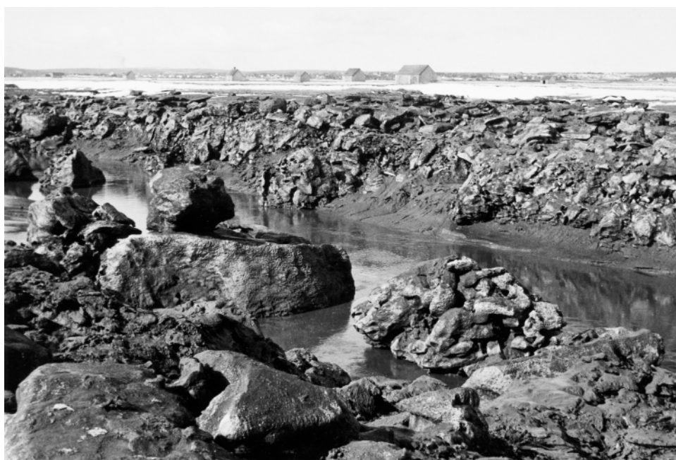
Fig. 51 Tantramar River between the C.B.C. transmitter and Middle March Road, about 2 km downstream from location shown in Fig. 50, 22 March, 1954. The tide is able to enter this section of the river (closed off by control gates about 1960) where an incomplete ice wall is formed. Ice block in right foreground is a conglomerate of many smaller ones. Left of centre, an ice block is stranded on top of another one, and frozen to it. Silt indicates that the ice was overtopped by the tide. Photograph #354-4.
