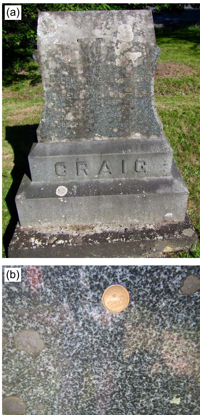
Figure 8. Monument for Joseph Craig (1830–1906), St. Andrews Rural Cemetery (a) Glenelg porphyry (diorite) headstone (b) Close-up of equigranular texture of the stone. Grey splotches are patches of lichen. Loonie coin for scale.
