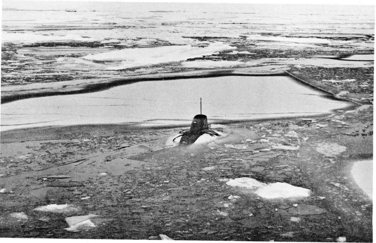
Figure 3 PISCES maneuvering in ice field before submerging. Submarine was tethered for traverses beneath ice cover but otherwise was free-diving. Photo by Dept. of National Defence.
