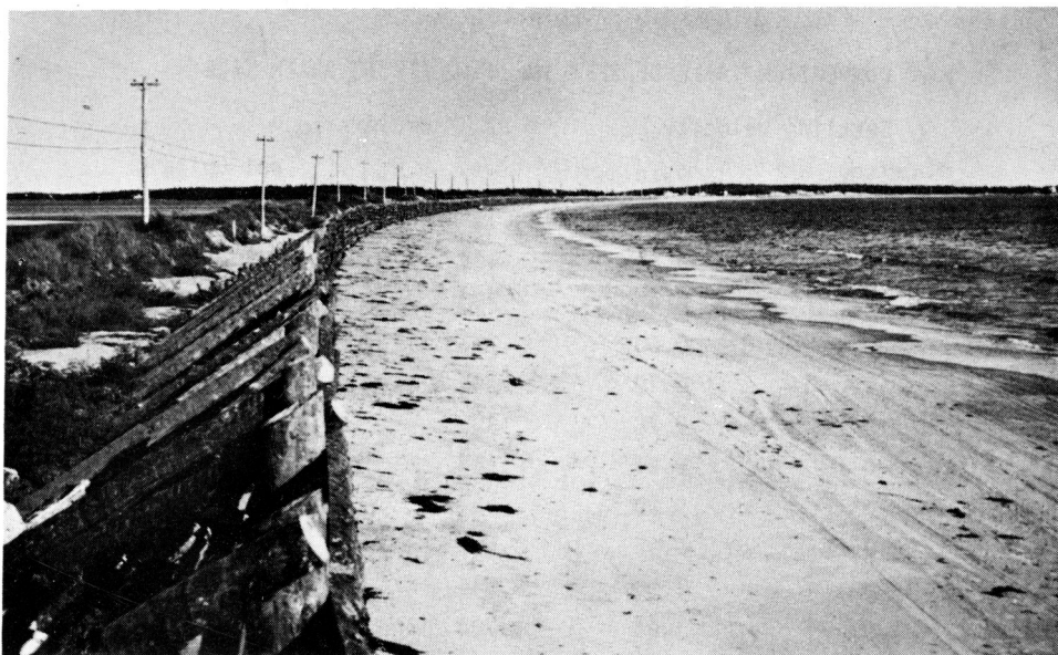
Fig. 5 - Green Bay foreshore.
