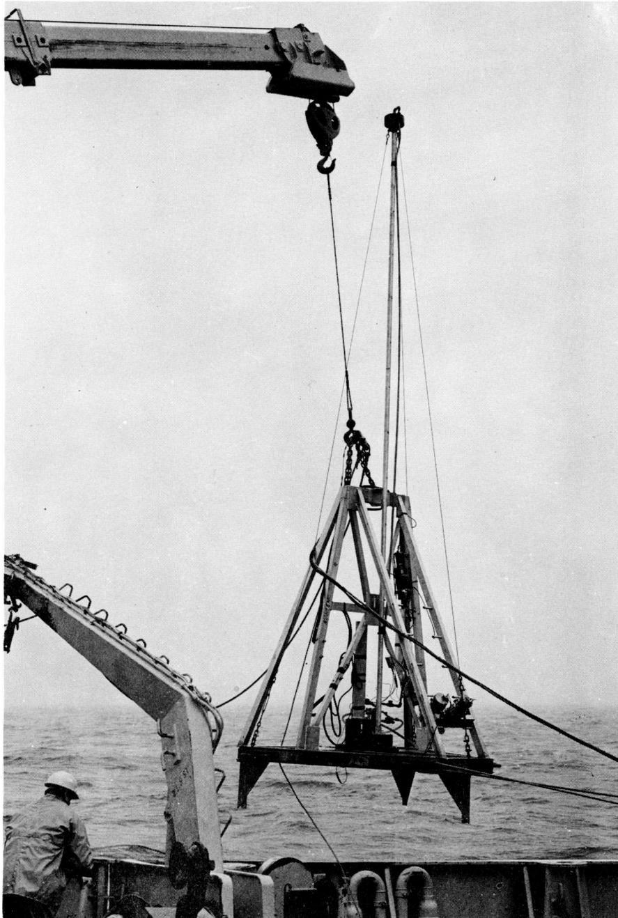
Underwater electric rock core drill developed at the
