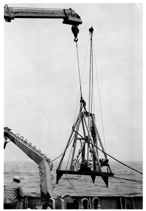
Underwater electric rock core drill developed at the Bedford Institute of Oceanography, Dartmouth, N.S.
