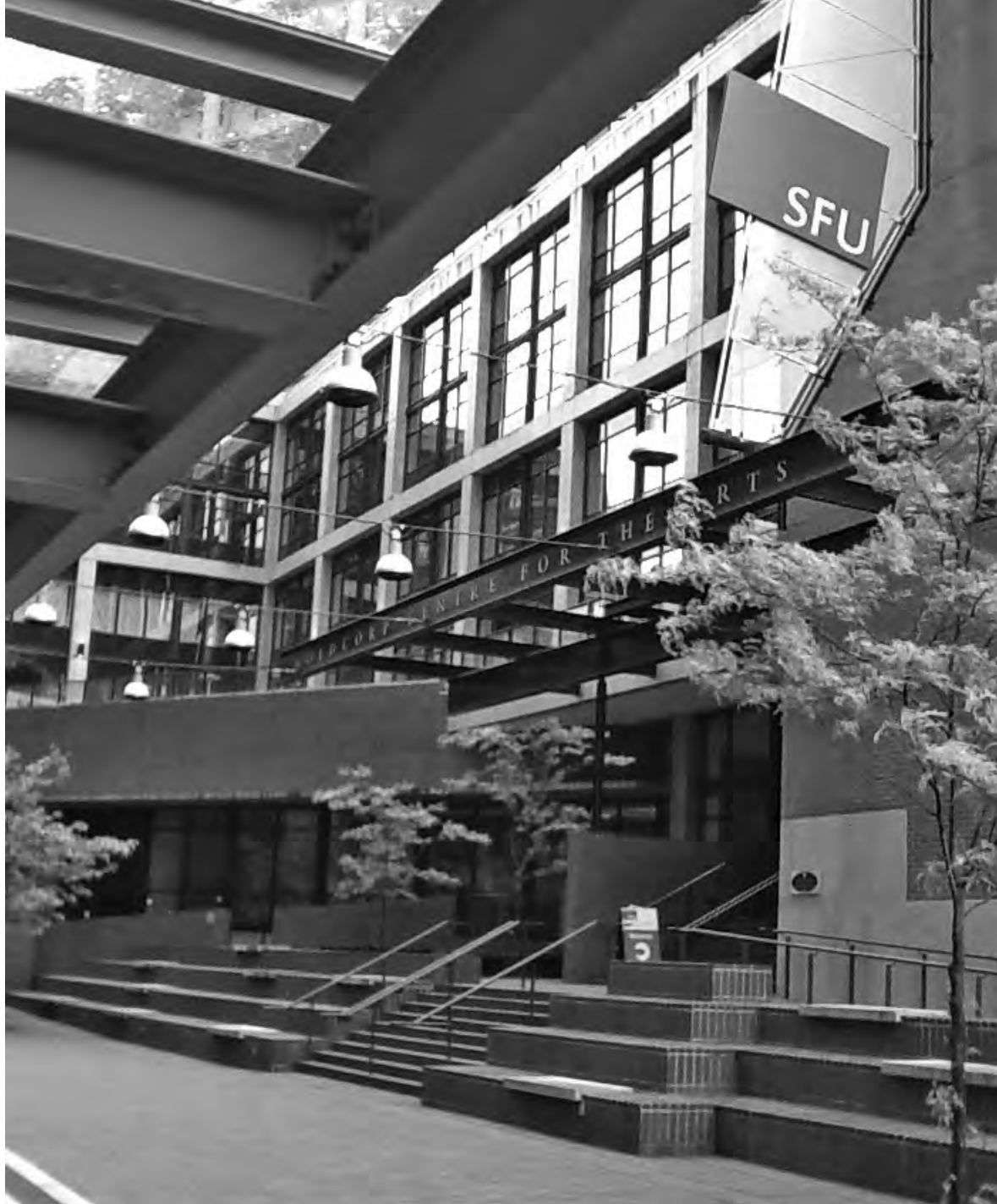
Figure 2. Entrance to SFU Woodward's via the Cordova Street atrium. Photo: Peter Dickinson.
