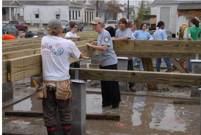
Rebuilding New Orleans.
