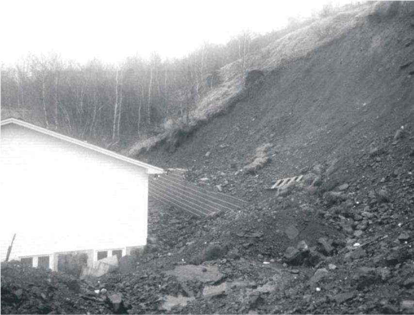
Figure 5. Recent construction on Southside Road, undercutting steep banks of till and increasing landslide hazard.
