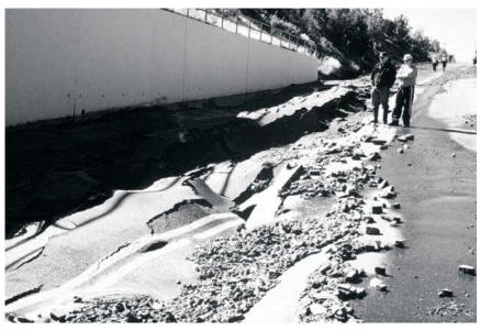
Figure 11. Flood damage on Shea Heights road, September 2001.
