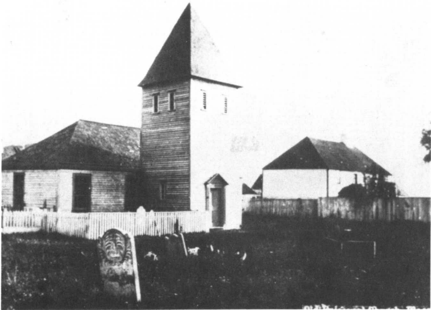
Pl. 1A: Anglican church (1787), cemetery and the courthouse at Placentia. The church and cemetery are on the same site as the French church, established by the Recollects in 1689, and used by the English after 1713.
