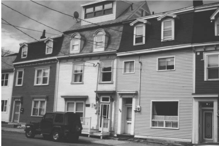
Figure 6. The discordant effect of inappropriate alterations on Gower Street.
