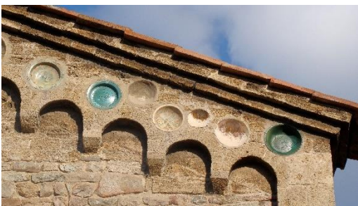
Figure 3 San Sisto, detail of bacini decoration on west façade. Photo by author.
