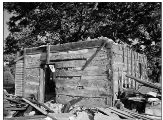
Fig. 19 (below) Henry Ronnebaum's one-room log house, St. Mary's Road, as it is being dismantled in June of 2010. Photograph by Gary Stanton.
