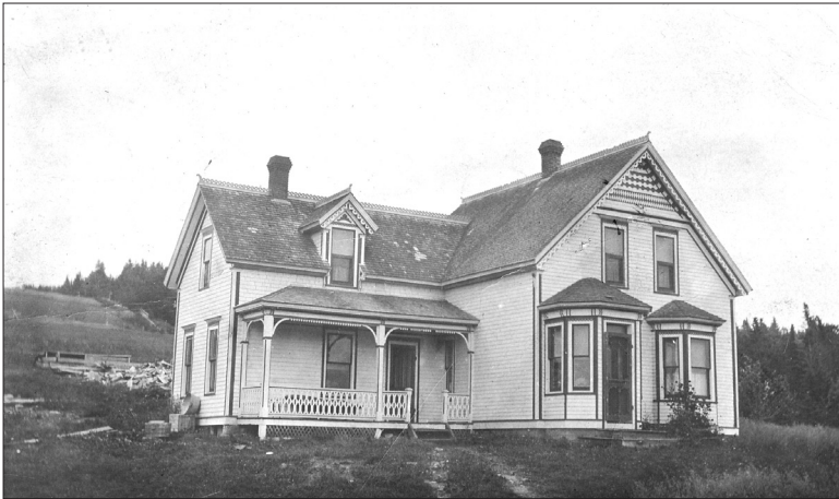
Fig. 23 (below) Isaac Fisher farmhouse, Fishers Mills, built in 1899. The house is built on a side-hall with integral kitchen ell plan. Note the application of machine-cut decorative trim and shingling, as well as the canted bay window and front door entrance. The building is more ornate than most St. Mary's domestic architecture. Photo courtesy Fisher family.
