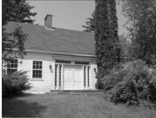
Fig. 5 (top) Countway-Mosher double house, Middle River, Chester Basin, Nova Scotia, built ca. 1839. Photo courtesy of the Heritage Division, Nova Scotia Department of Tourism, Culture and Heritage, 2007. Available from https://www.historicplaces.ca/en/rep-reg/place-lieu.aspx?id=9086 .
