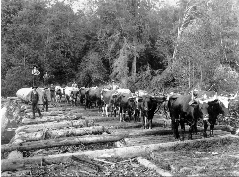
Fig. 4 Logging with oxen on a corduroy road; the Brunette Sawmill Company's logging team on the Nicomikl River, ca. 1870. Source: Royal BC Museum and Archives, C00570. The two large logs are about to be rolled into the river where others can be seen at the edge of the photograph.
