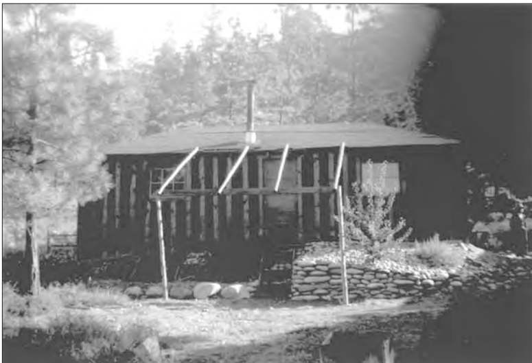
Fig. 1 "1943 May. Matsui House clad with tar paper to be wind proof. The only house with a basement." 2 Image courtesy of the Japanese Canadian Cultural Centre, 2011.47.06.06.15.
