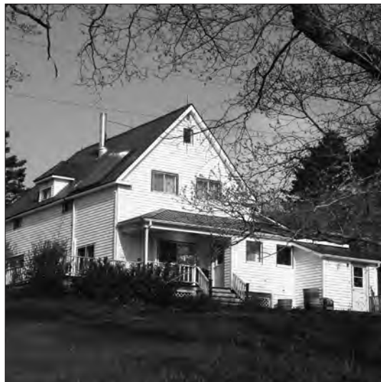
Fig. 10 Archibald farmhouse, ca. 1915. Various porch additions and extensions to the façade are visible. Photo by author.
