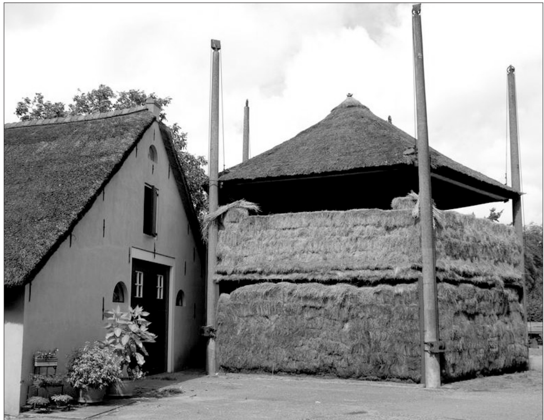
Fig. 3 Four-pole hooiberg with pulleys at Franschepad, Blaricum, Netherlands. (Photo courtesy Gerard Grootveld.)
