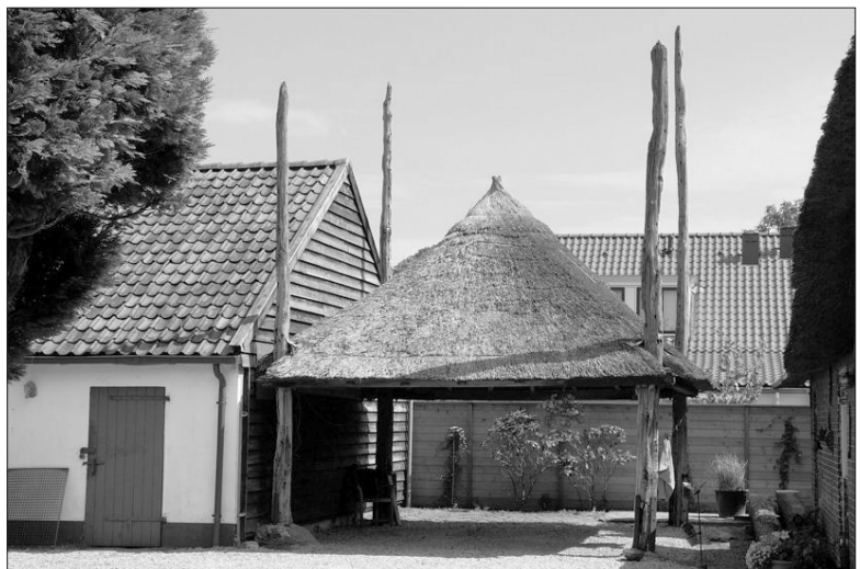
Fig. 2 A ca. 1930s four-pole hooiberg at Emnesserweg, Blaricum, Netherlands. (Photo courtesy Gerard Grootveld.)
