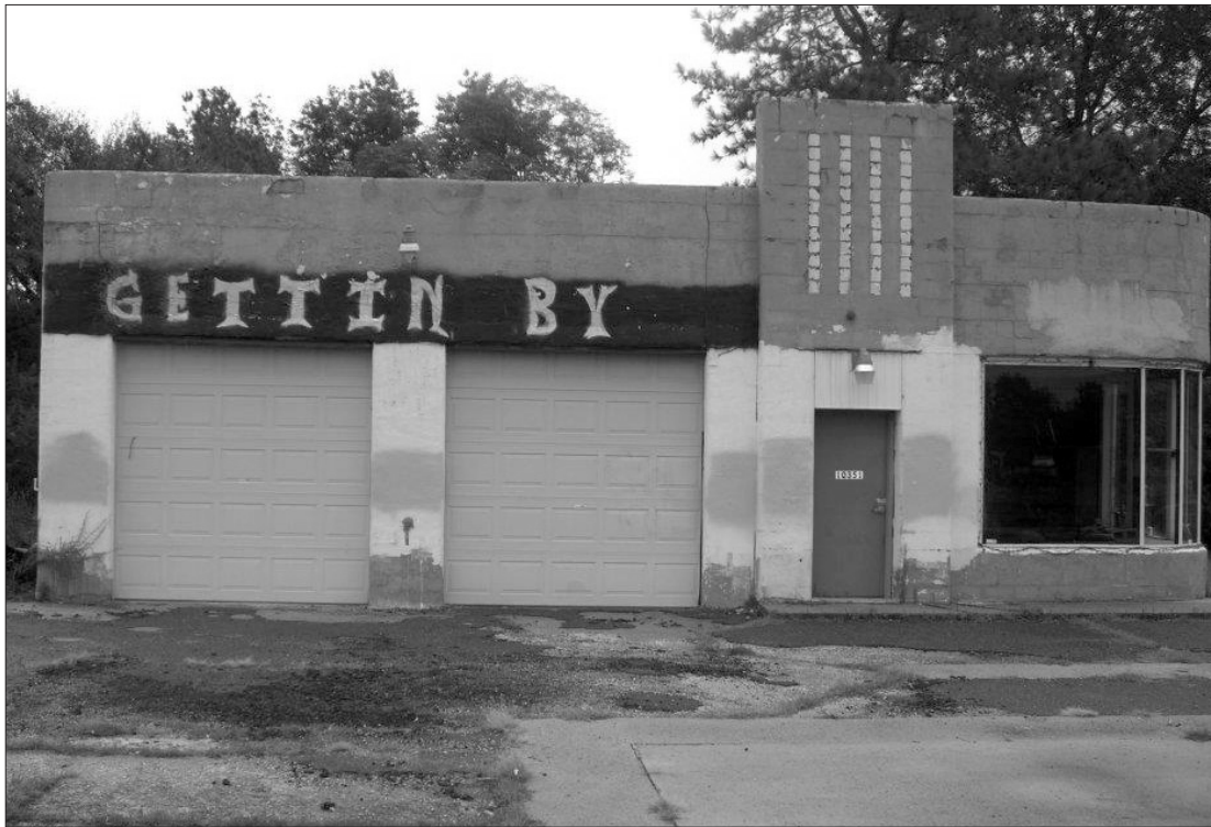
Fig. 3 This former gasoline station is currently abandoned and sitting derelict. (Photo by authors.)
