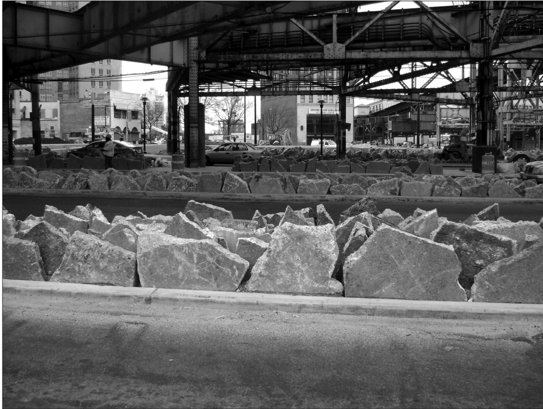
Fig. 12 The functional reuse of waste concrete captures and creates value, while also animating the narrative by exposing marks from previous use and demolition. Photo by author.
