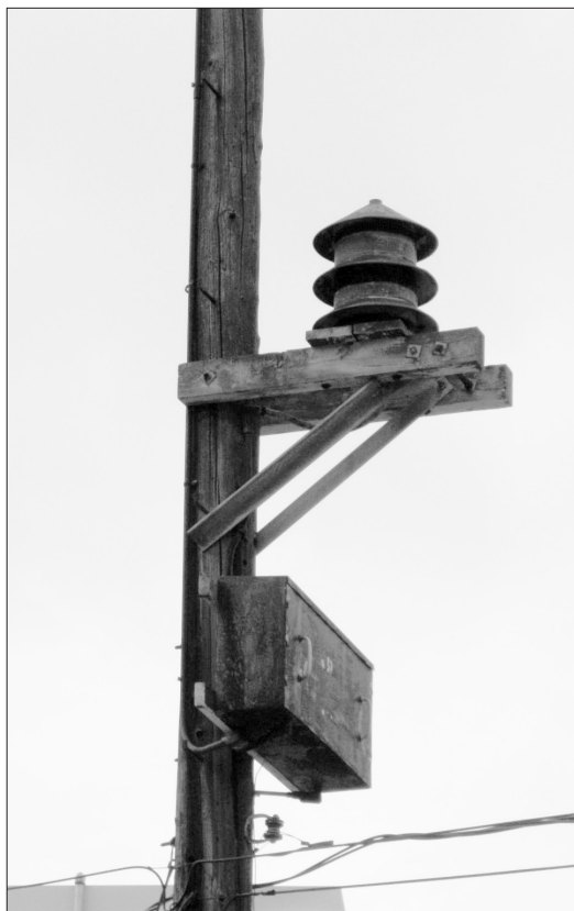
Fig. 2 A two-horsepower Federal siren, installed on a hydroelectric pole in Welland County, Ontario. Courtesy of Mark Reesor.
