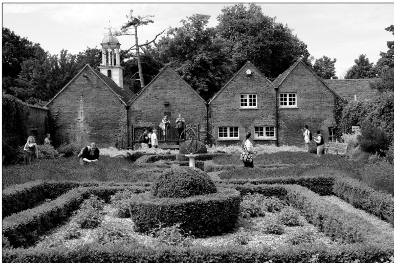
Fig. 2 The Museum of Harlow is located in the former Mark Hall stable block (ca. 1785). Photo: Gerald Pocius.
