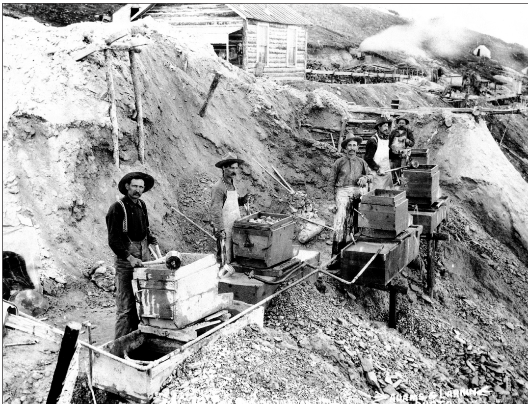
Fig. 6 Miners rocking for gold on Klondike hillside ca. 1900. Note the dippers being used to pour water. Yukon Archives 3928.
